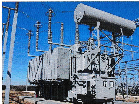
Electrical transformer with surge arresters on top
